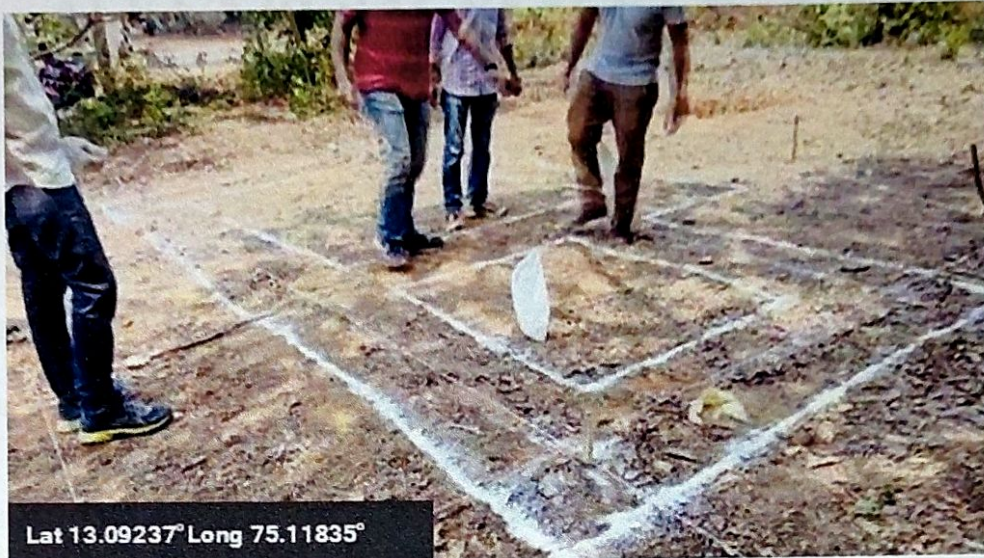
Foundation Marking for Toilet Complex
