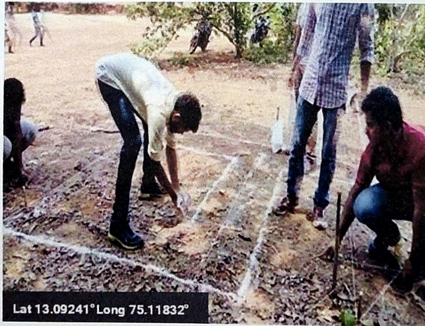
Students Marking Foundation for Toilet Complex
