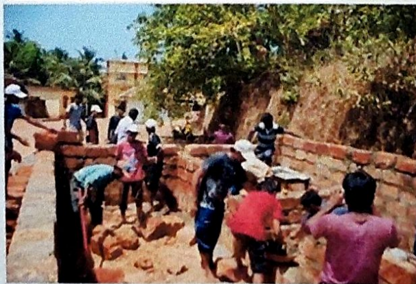
Construction of Footing
