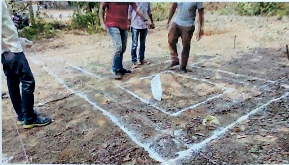
Foundation Marking for Toilet Complex
