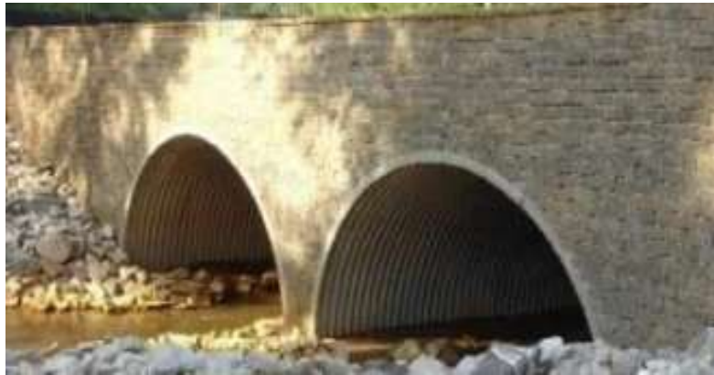
Fig.2.1.7 Pipe Arch Culvert
