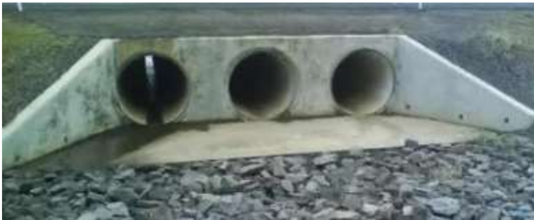
Fig.2.1.6 Pipe Culvert
