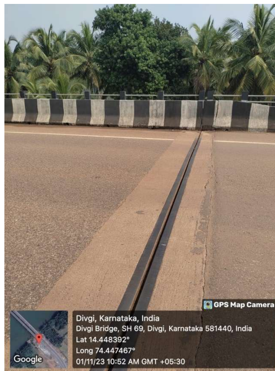
Fig 2.1.5 Expansion Joint
