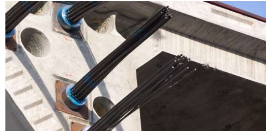
Fig: 2.1.4 Prestressed Cable
