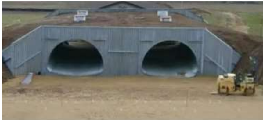
Fig.2.1.9 Arch Culvert
