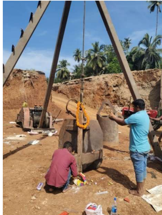
Fig 2.1.14 Pile Boring Machine
