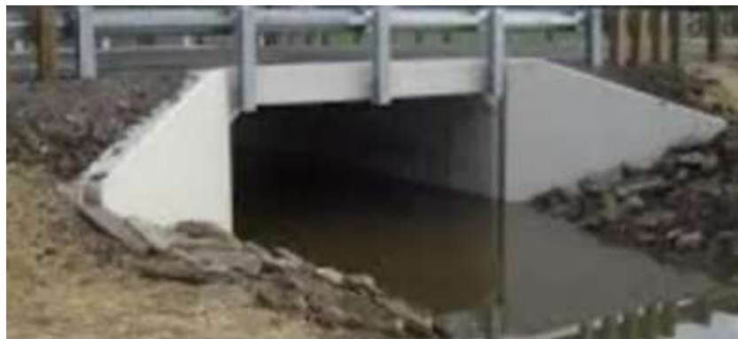
Fig: 2.1.10 Bridge culvert
