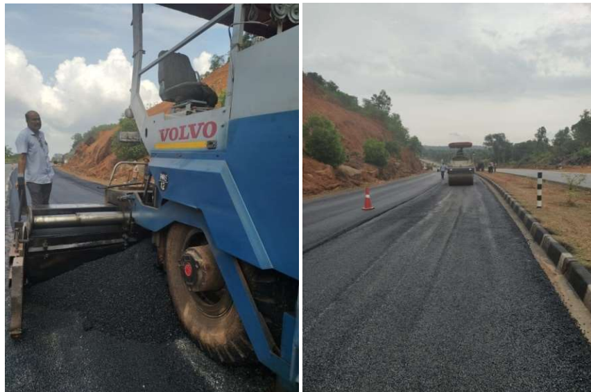
Fig.2.2.9 Laying BC layer with Paver
