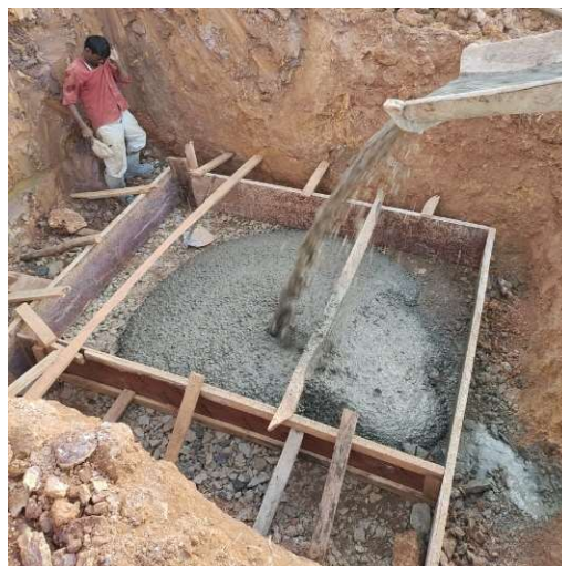
Fig 2.1.18 PCC laying
