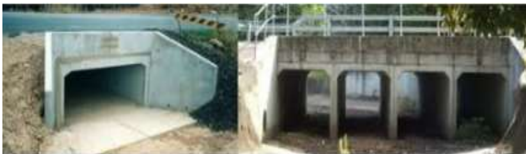
Fig.2.1.8 Box Culvert
