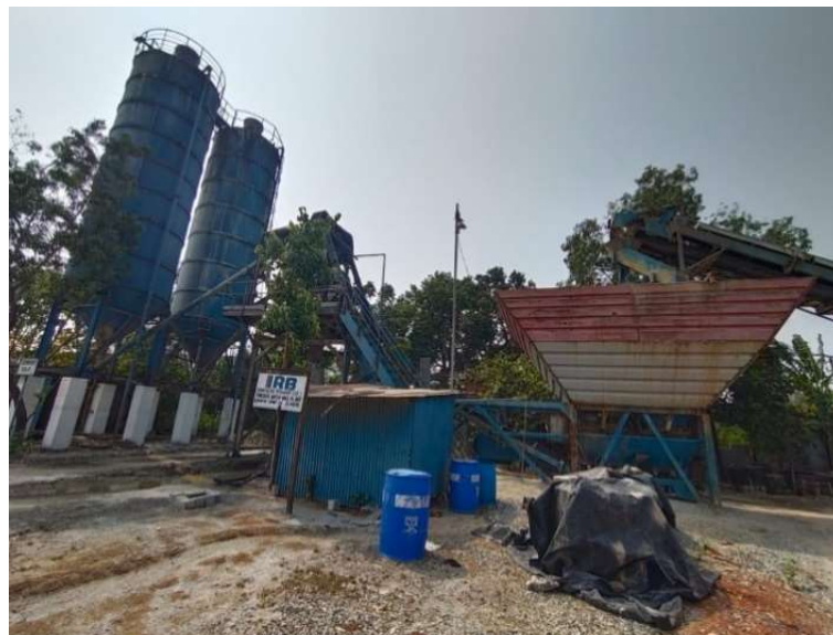
Fig 3.14 Ready Mix Concrete Plant
