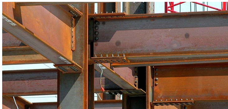
Fig.5 Moment connection
