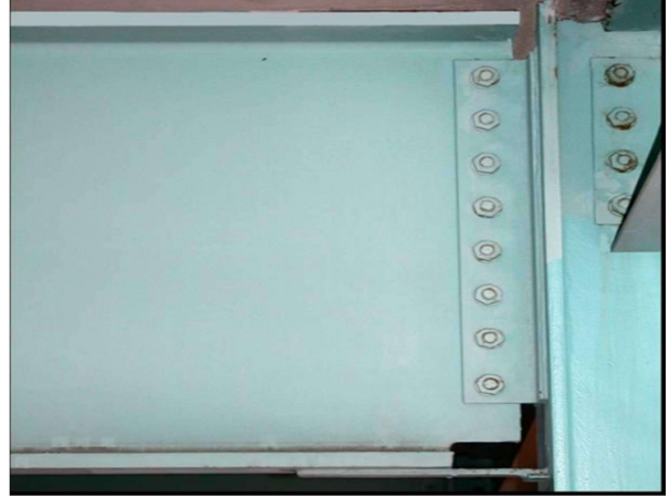
Fig.7 Partially restrained connection
