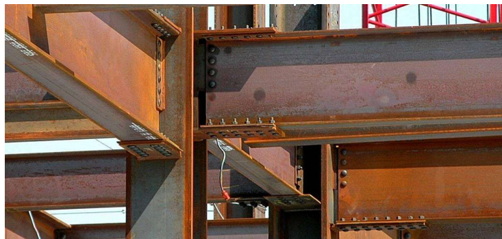
Fig.5 Moment connection
