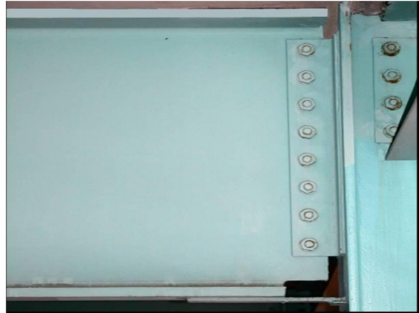
Fig.7 Partially restrained connection
