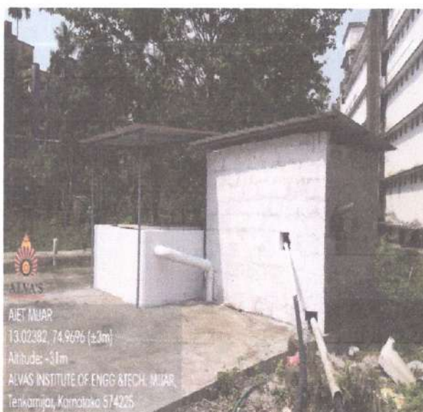
Treatment Chamber of Size 3m x 2m x 1m
